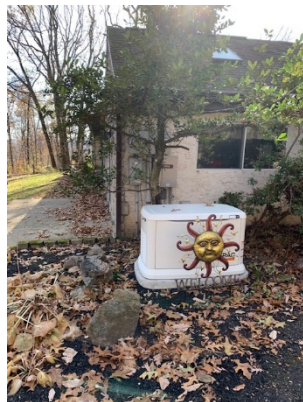
Before and after pictures of the generator installation at Alaina's home.
